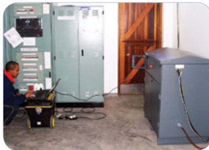
The Pnu Power 5™ (above centre) provides reliable standby power for a critical switchboard which is part of Eskom's Cape Town electricity distribution network.
