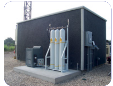
The Pnu Power Compressed Air Battery installation at Brooksville features a 300 Bar (4350 PSI) air store with auto recharge compressor.
