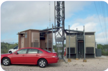
The Pnu Power Compressed Air Battery installation at Brooksville features a 300 Bar (4350 PSI) air store with auto recharge compressor.
