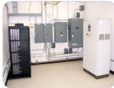
The Pnu Power Compressed Air Battery installation at Brooksville features a 300 Bar (4350 PSI) air store with auto recharge compressor.
