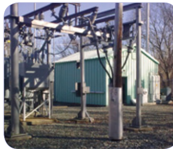
The Pnu Power Compressed Air Battery at Barrington on Rhode Island is installed externally and is totally weatherproof.
